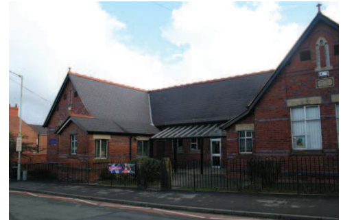
Slate Gable Roofs
